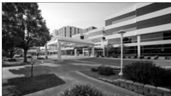
BryanLGH Medical Center WEST
